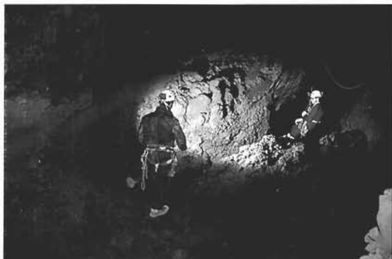
Fig. 5 - Small room generated by collapsed walls.
